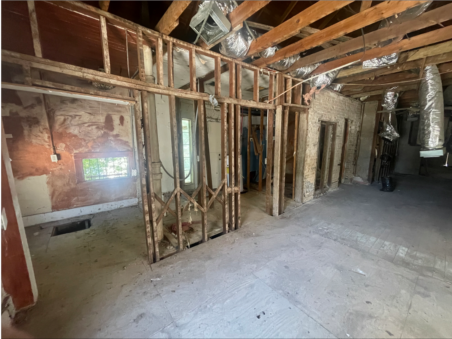
Interior shell ready for finish out
