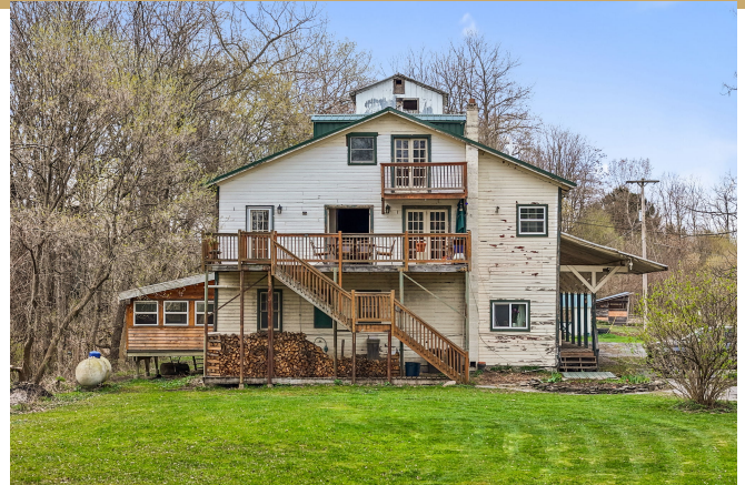
Rear elevation showing residential apartment and porch
