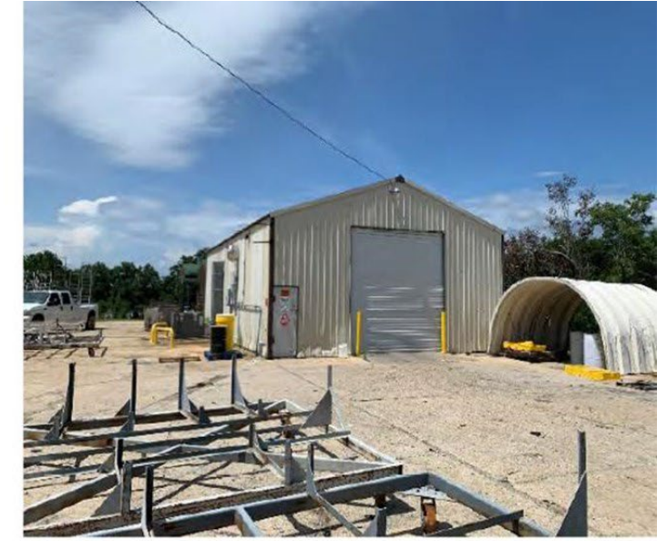
CHEMICAL STORAGE BUILDING
