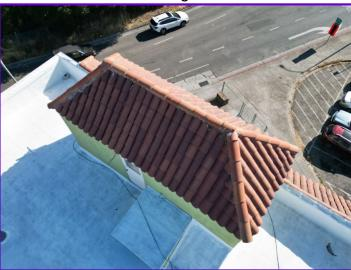
COMMENTS: The composite tile roofing material COMMENTS: The composite tile roofing material appears to be in satisfactory condition relative to its age.
