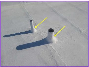
PREVENTIVE: The plumbing vent protrusions appeared to be properly flashed but lacked storm appeared to be properly flashed but lacked storm collars.
