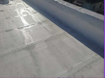
MONITOR: Water stains were noted in areas of the flat roof. This indicates water has pooled in the past and will likely continue to pool.
