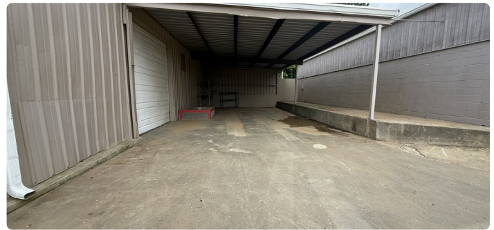
Covered canopy / dock area
