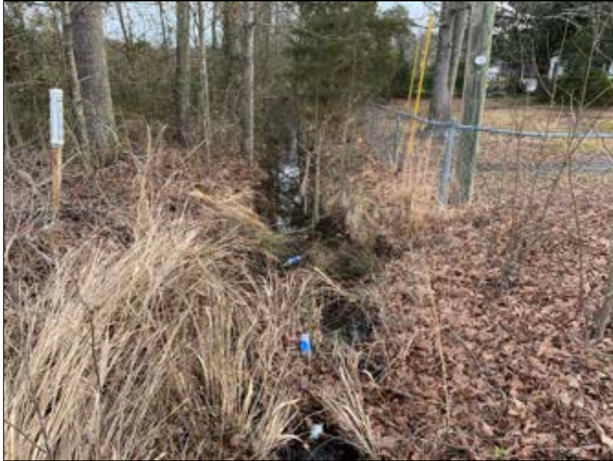
19 - View of the drainage ditch/creek that presumably forms a portion of the Property's southern border.
