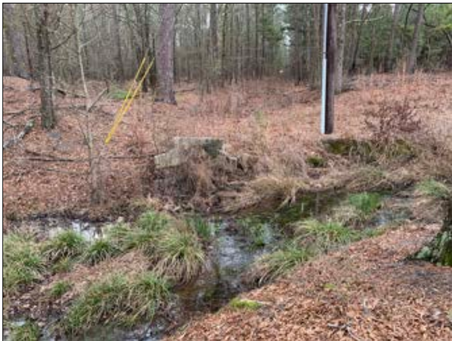
20 - View of the Property's eastern corner. The concrete embankment signifies off-site run-off being directed toward the streams bordering the Property.
