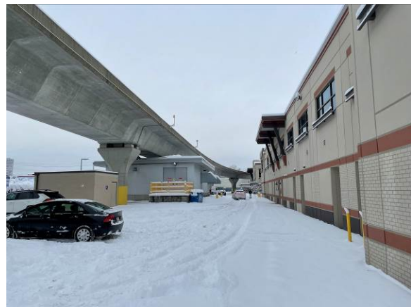
View of Parking, Guideway, and Rear
