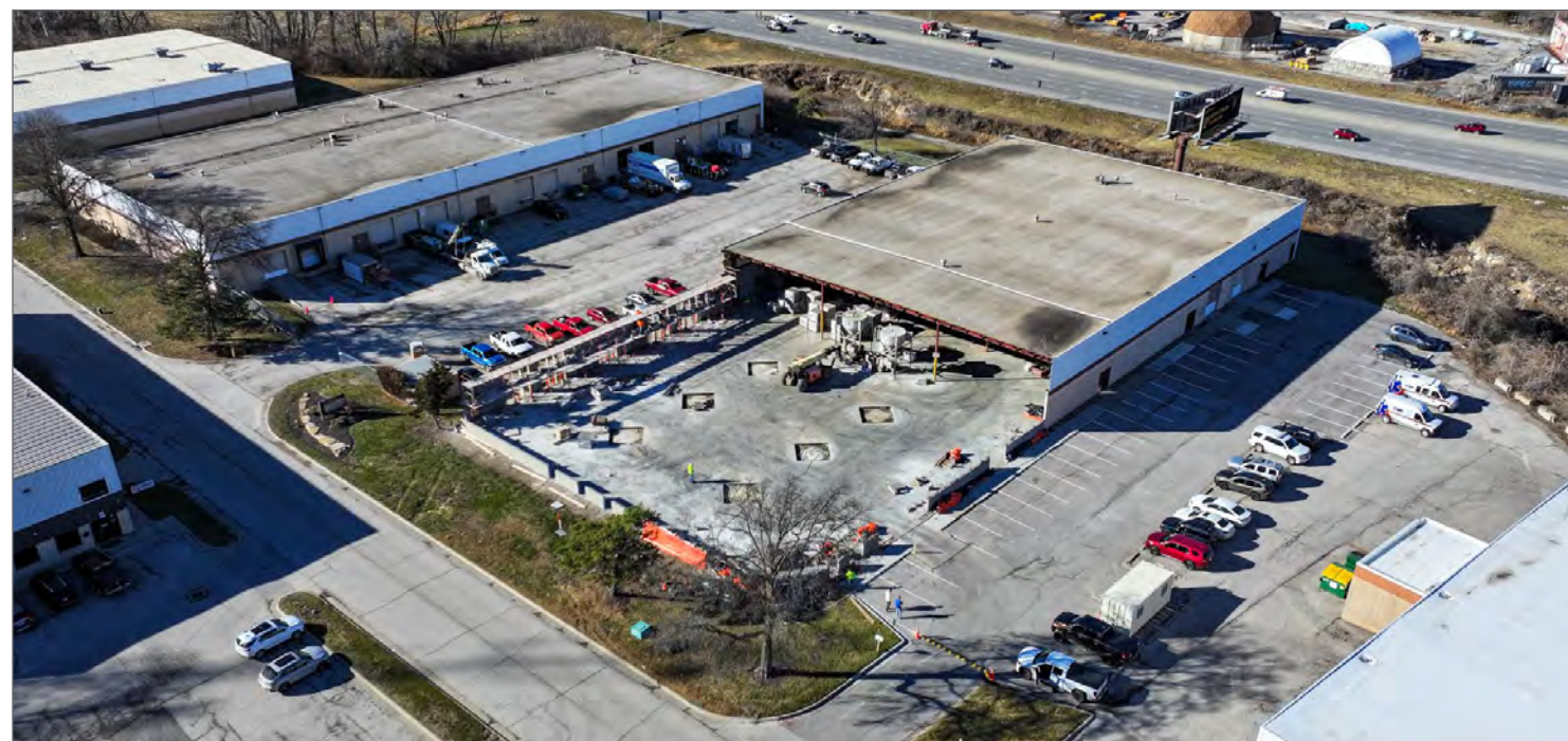
Photos of new construction in progress January 2026.
