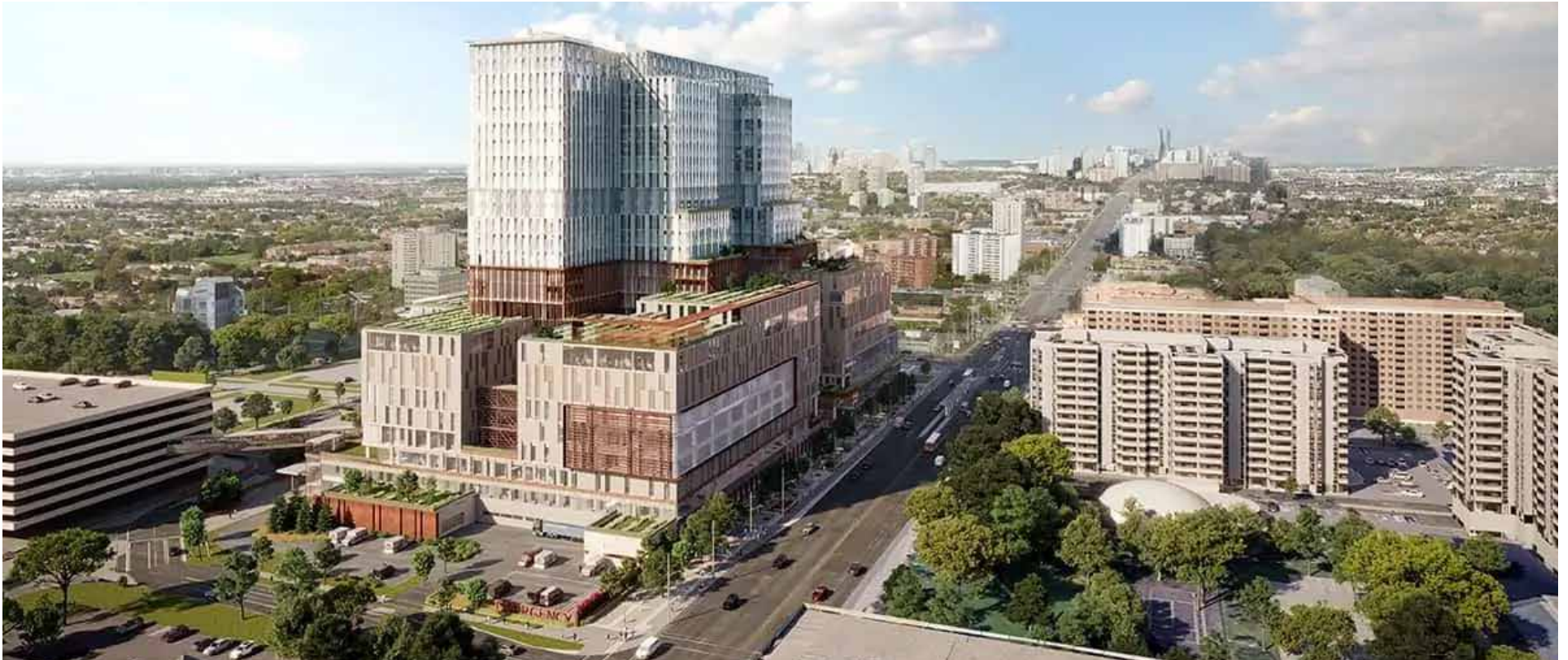
The new 24-storey Mississauga Hospital, when completed, will be among the largest hospitals in Canada.
