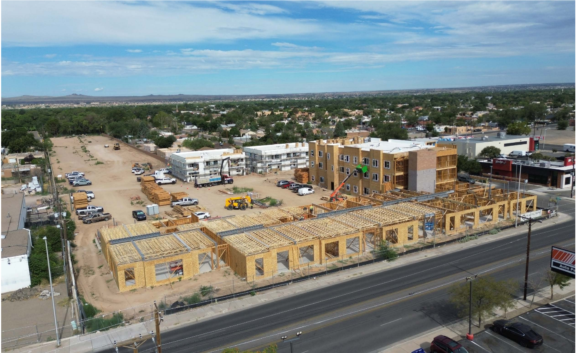
Construction Progress as of August 2024
