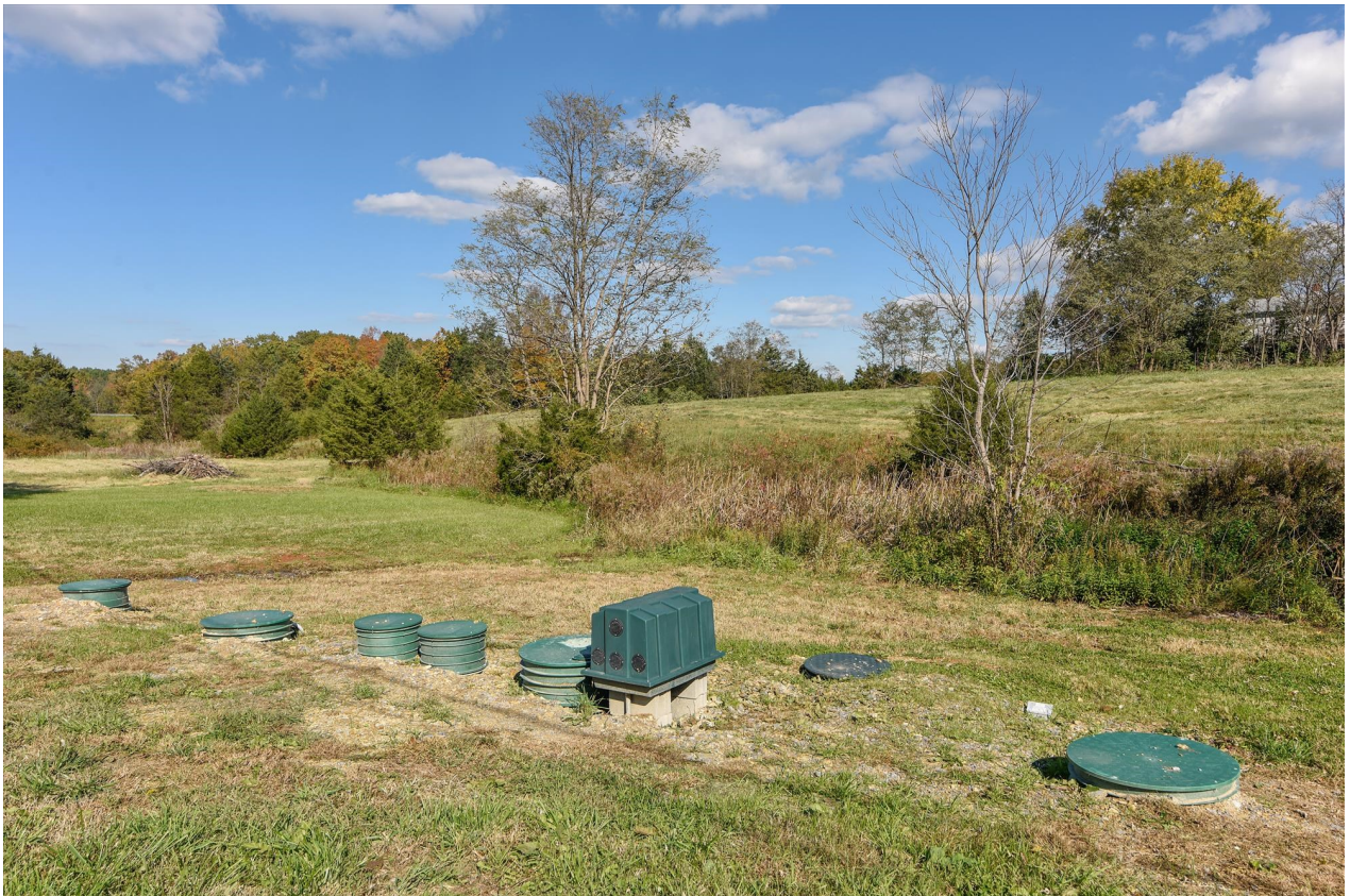
New Septic System
