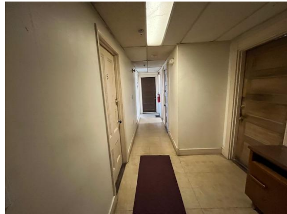
1 st floor common area
