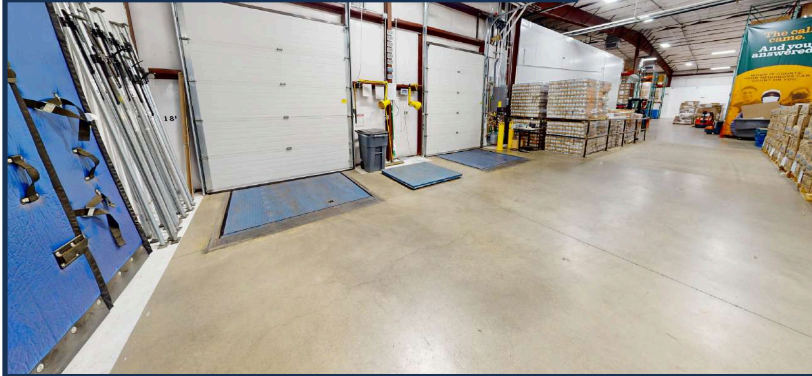
Dock-High Doors With Levelers
