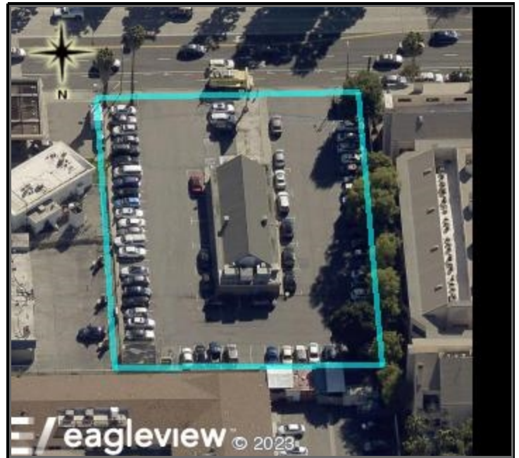
View Looking South
