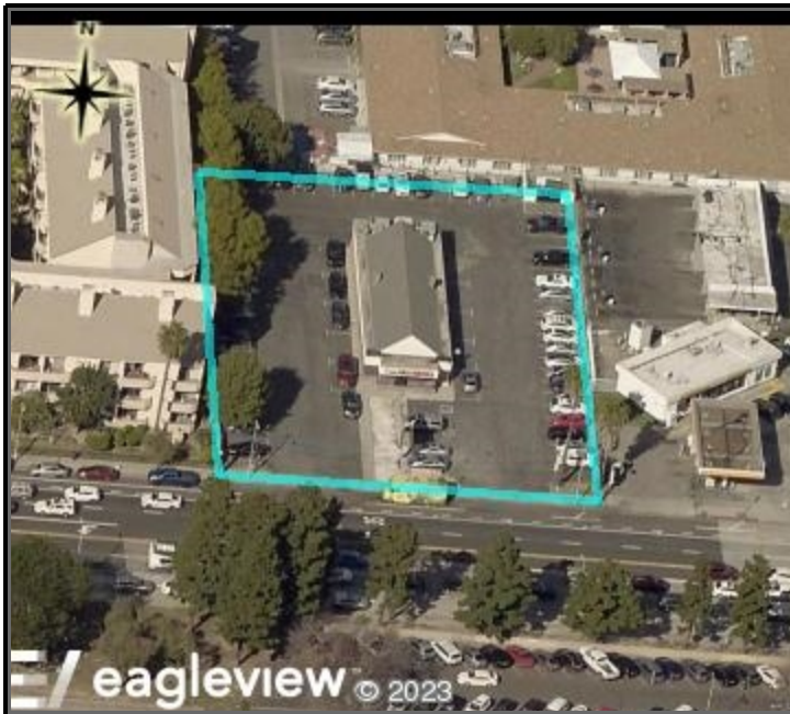
View Looking North
