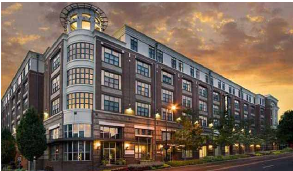
Figure 2.8: Example of residential and streetscape
