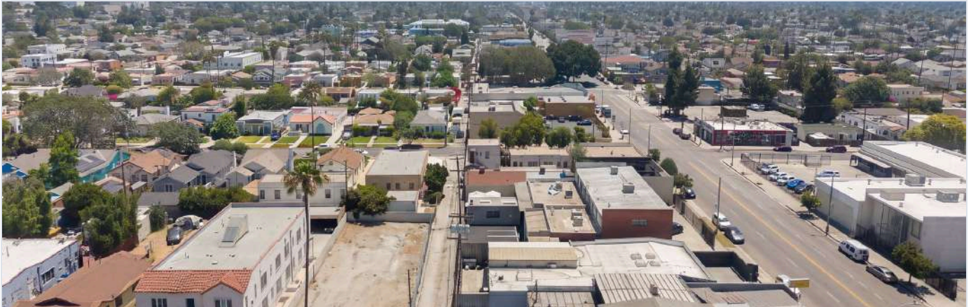
THE RESTAURANT CORNER WITH ITS DEDICATED REAR PARKING LOT AT 3050 EDGEHILL DRIVE — ±26 STRIPED SPACES ON FEE-OWNED LAND
