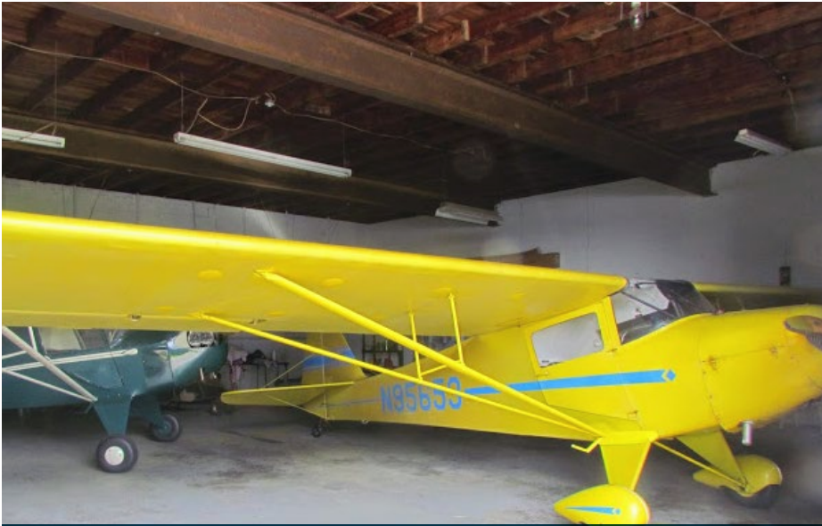
Inside of concrete hanger built originally for Beechcraft King Air planes
