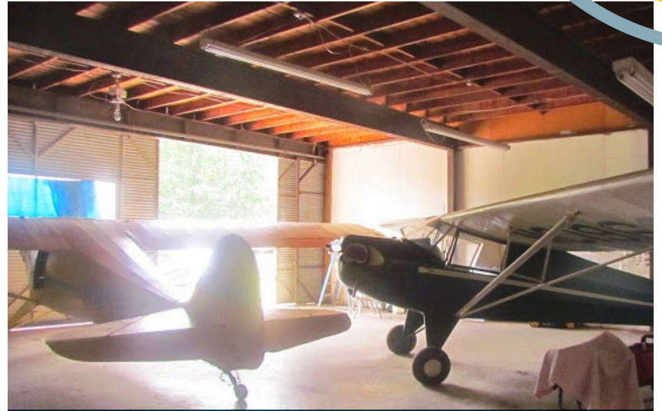
Inside of concrete hanger built originally for Beechcraft King Air planes
