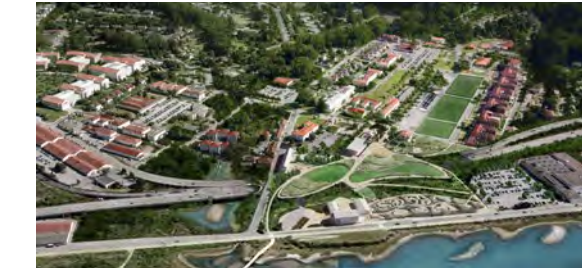
PRESIDIO TUNNEL San Francisco
