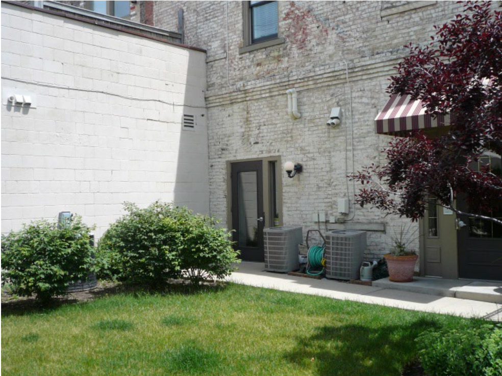
Main Residential and Limited Commercial Condo Lobby Entry
