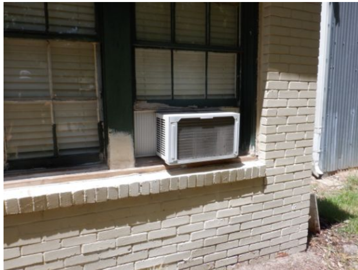
Note: Window units are not inspected.
