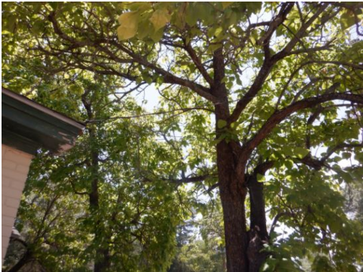
Recommend the trees be trimmed away from the overhead electrical service lines.
