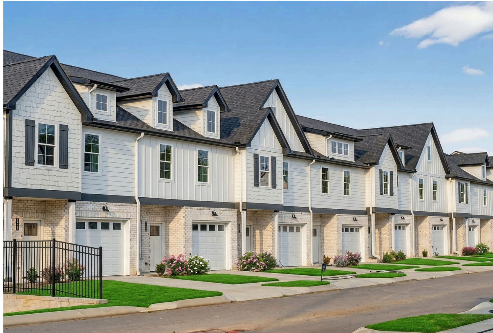
2024-built townhome community · Lebanon, TN
