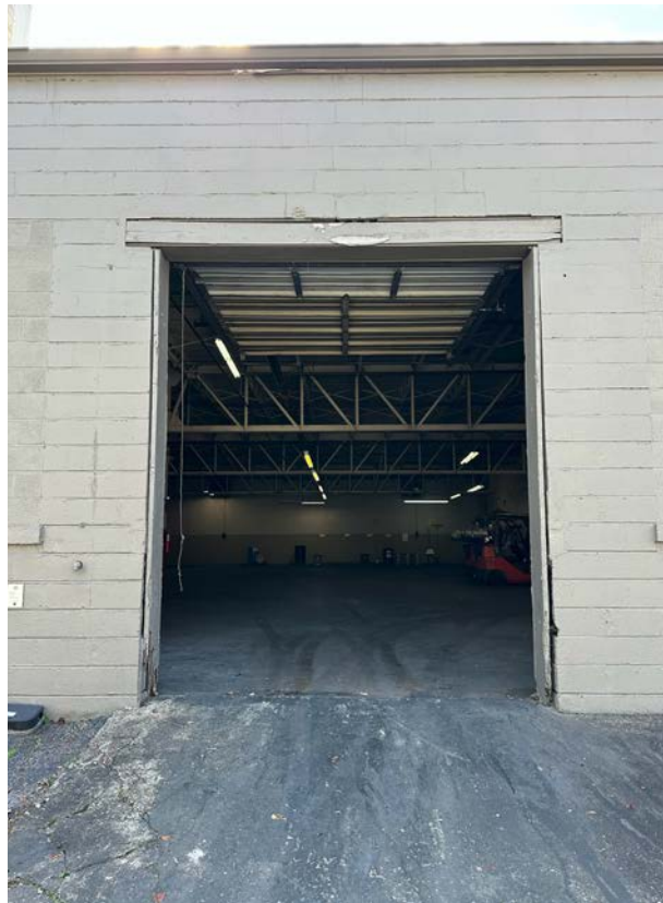
Drive In Overhead Door
