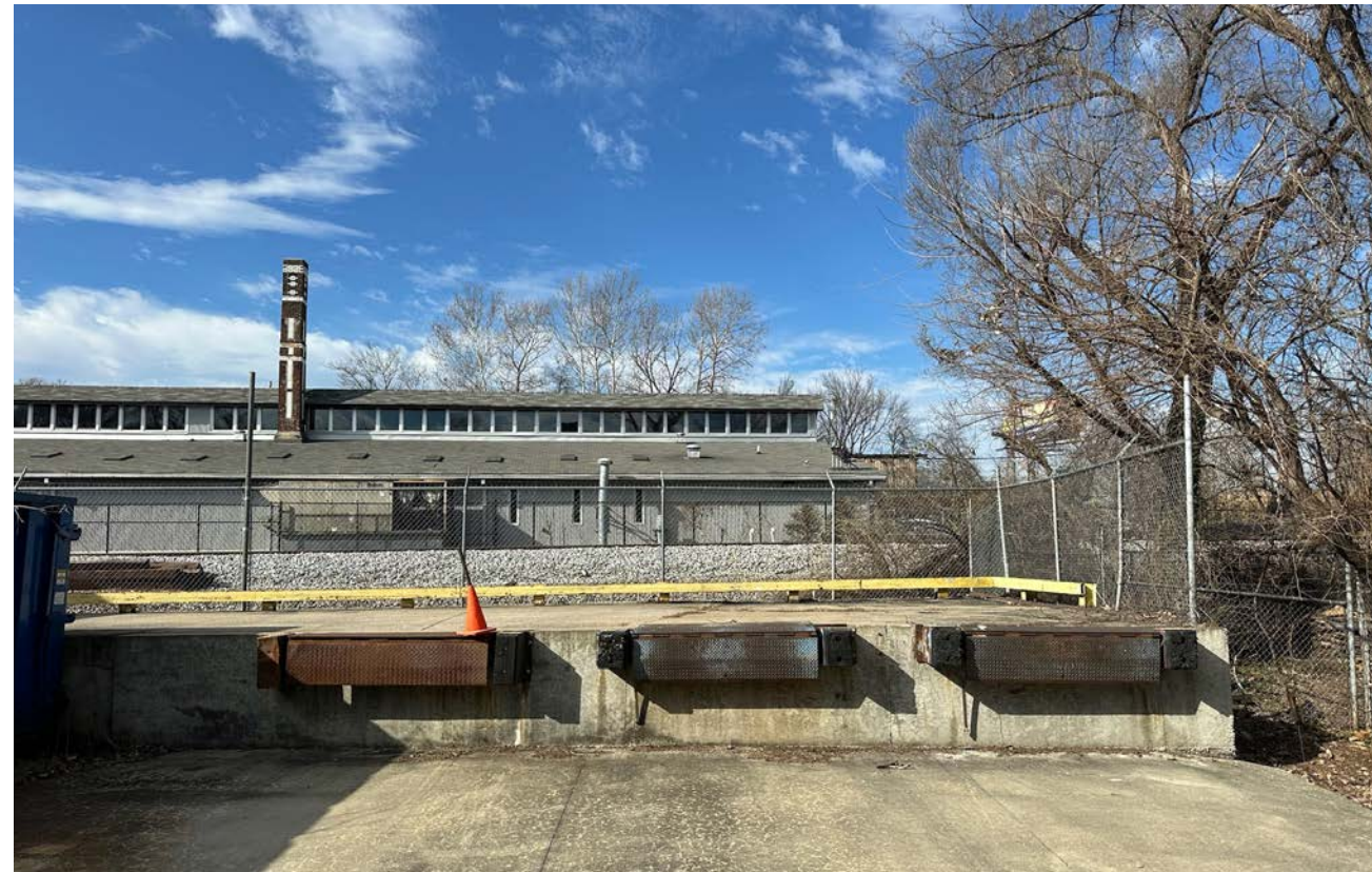
Loading Platform Positions w/Levelers
