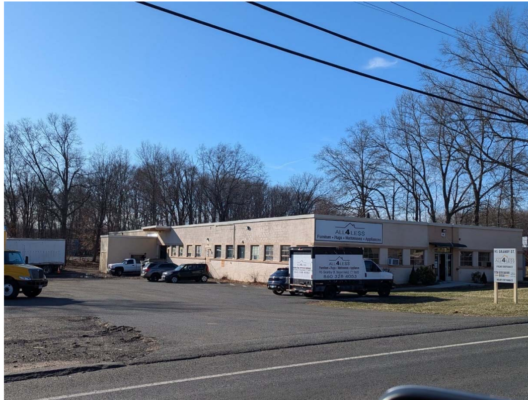
Subject Property – Front of Building – View West
