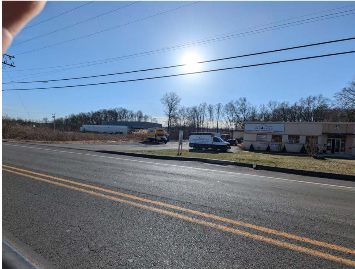
Subject Property – New Roof and Solar
