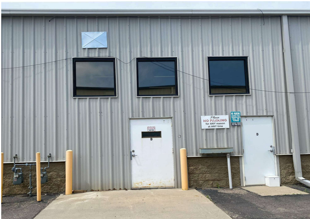
Two rear doors to unit production area, potential for 9' - 10' wide overhead door with 8' - 14' height
