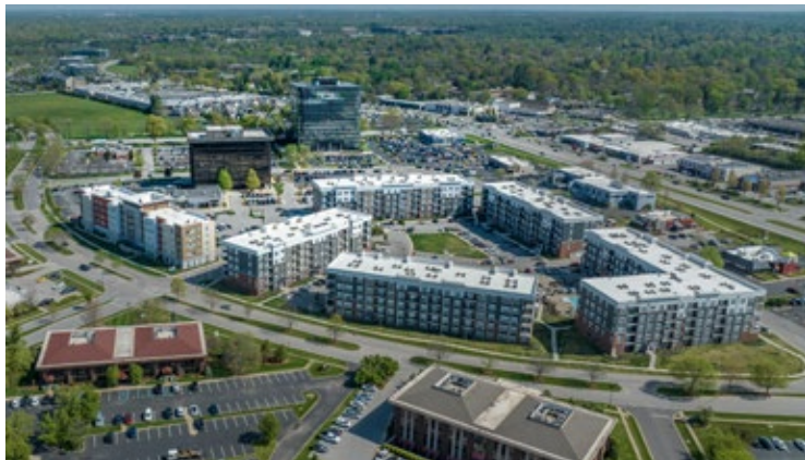
Adjacent to the newly-constructed Rialto Hurstbourne apartments
