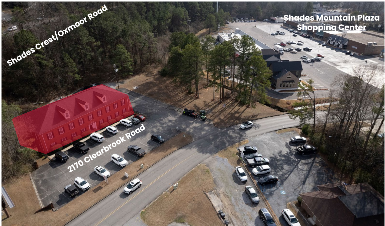
Rear Parking Lot
