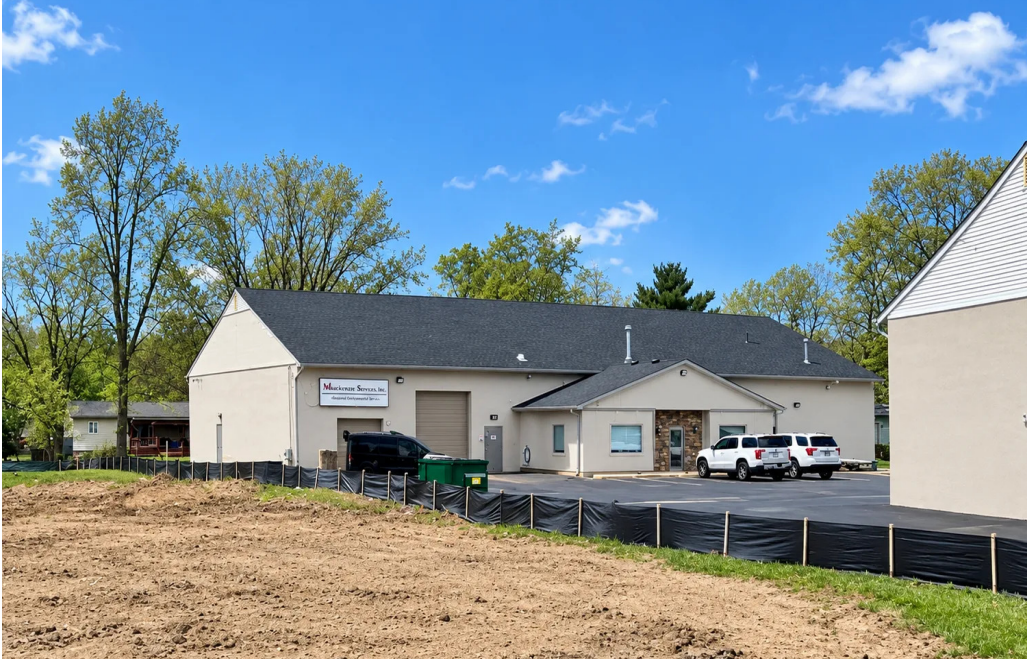
BUILDING #1 - 9897 Weber Street (Back Building) - 9,180 SF
