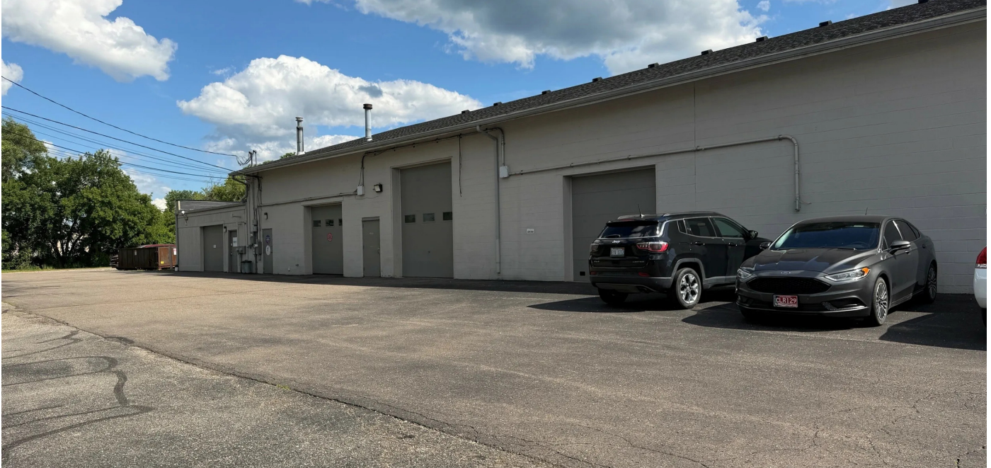
BUILDING #2 - Rear Building Photo
