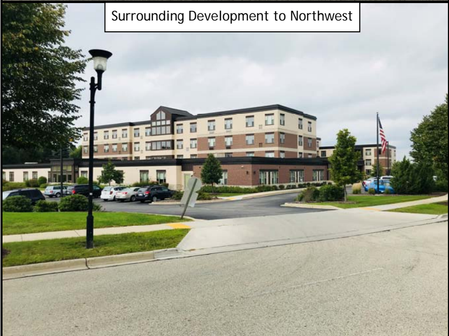
Surrounding Development to Northwest
