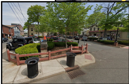
Front View from Ferry/Kline corner
