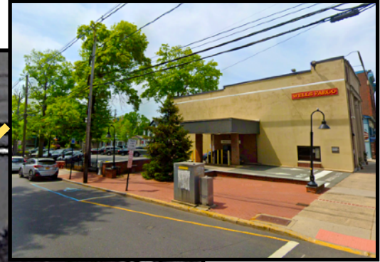
Side View from Bridge Street
