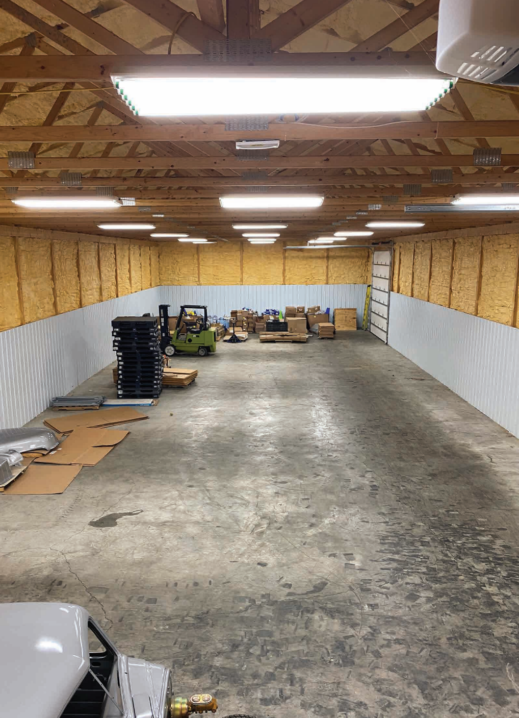
Building 247: Open Warehouse View from Mezzanine.
