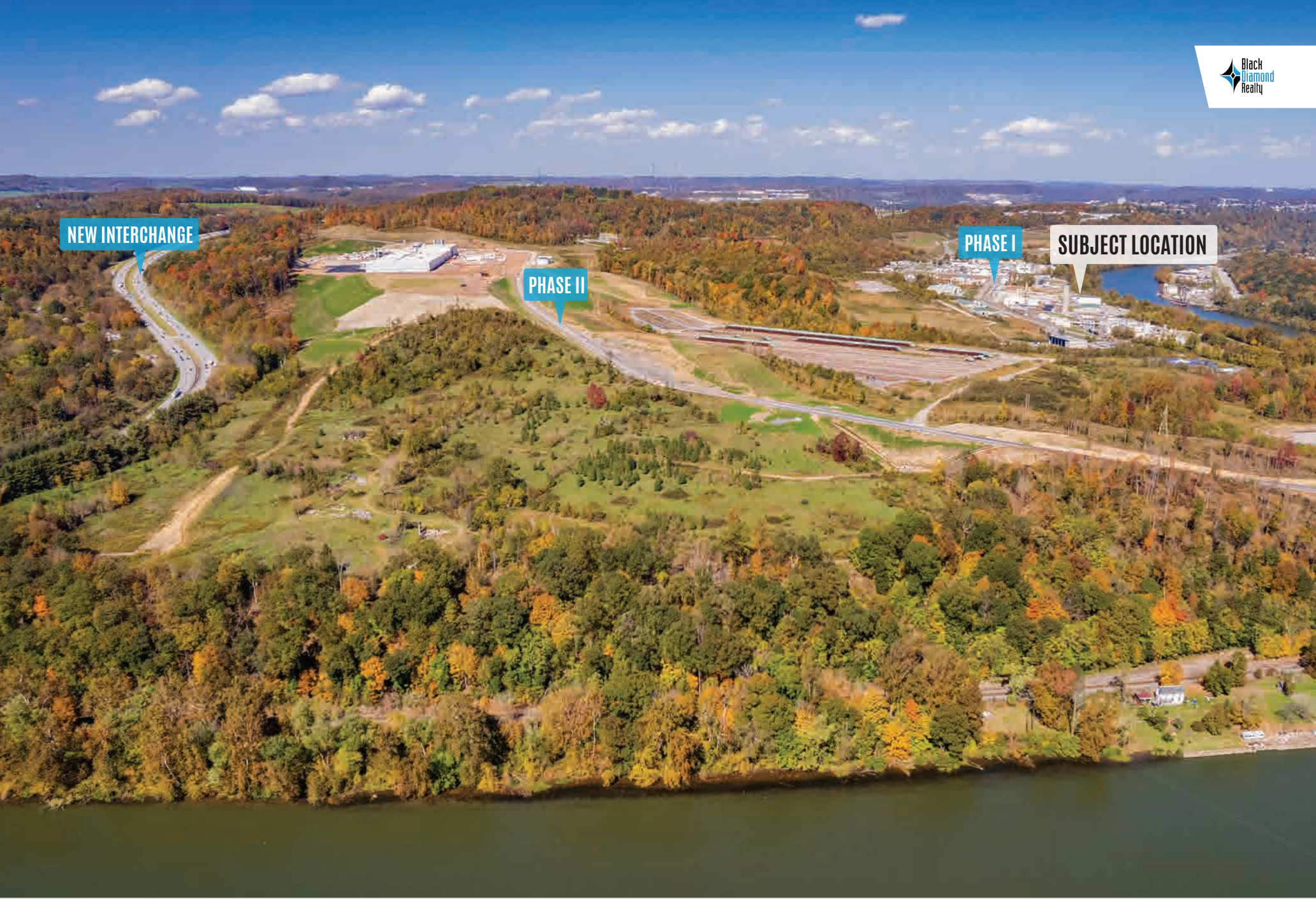
Aerial of Phase I and II Facing North.
