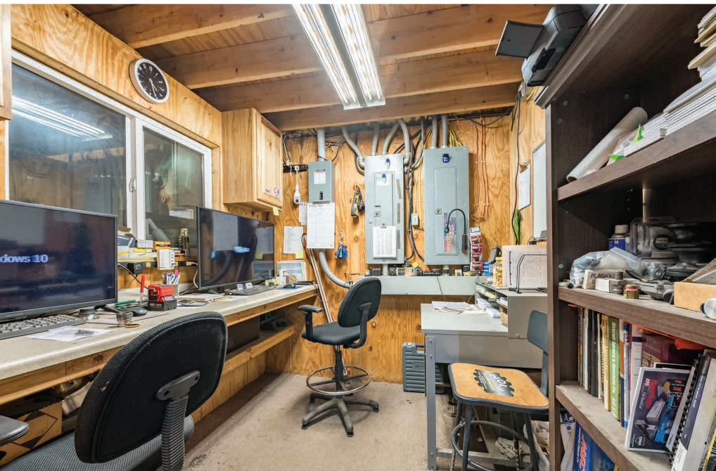
Industrial Area Office.
