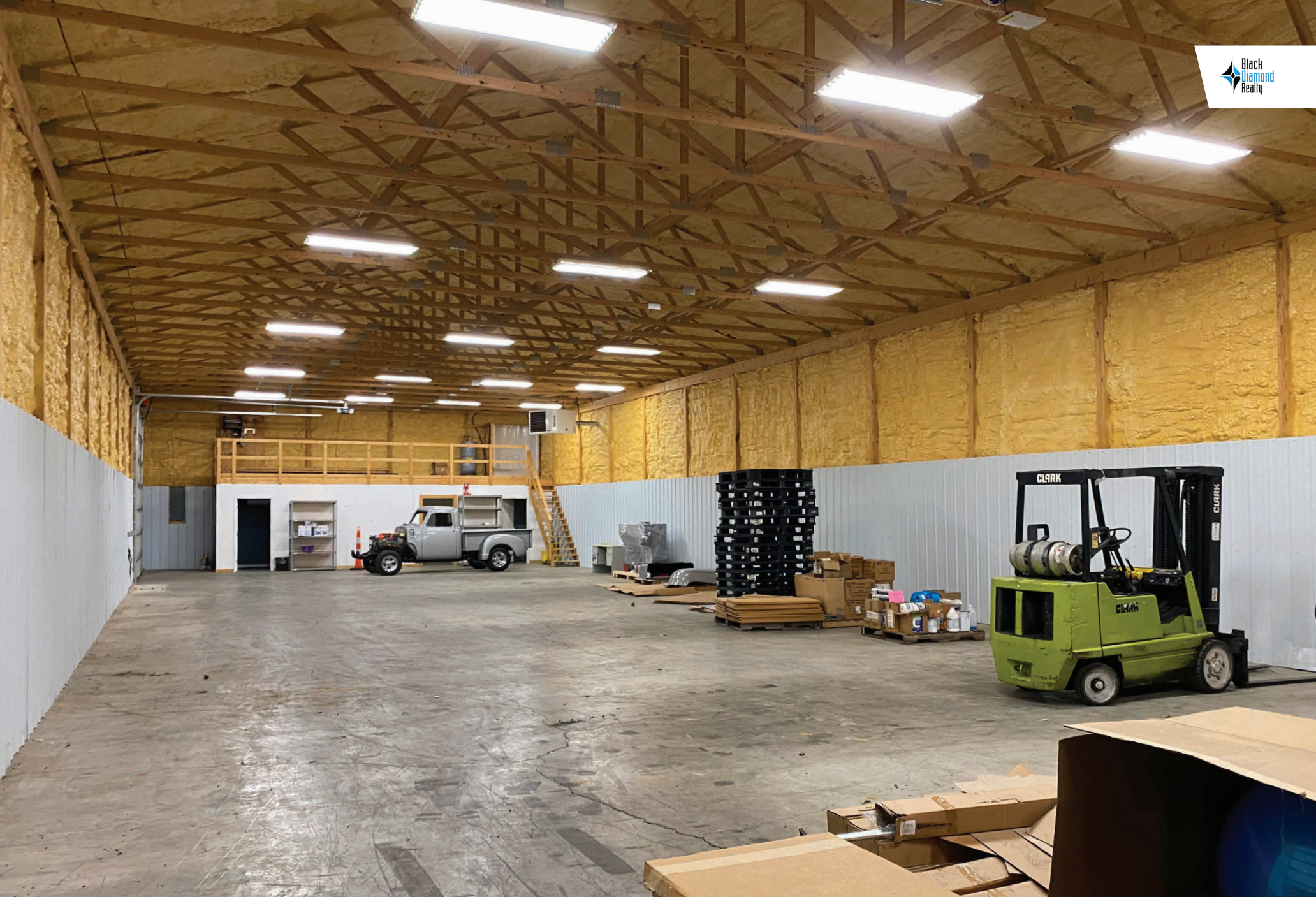
Building 247: Open Warehouse Facing Mezzanine.
