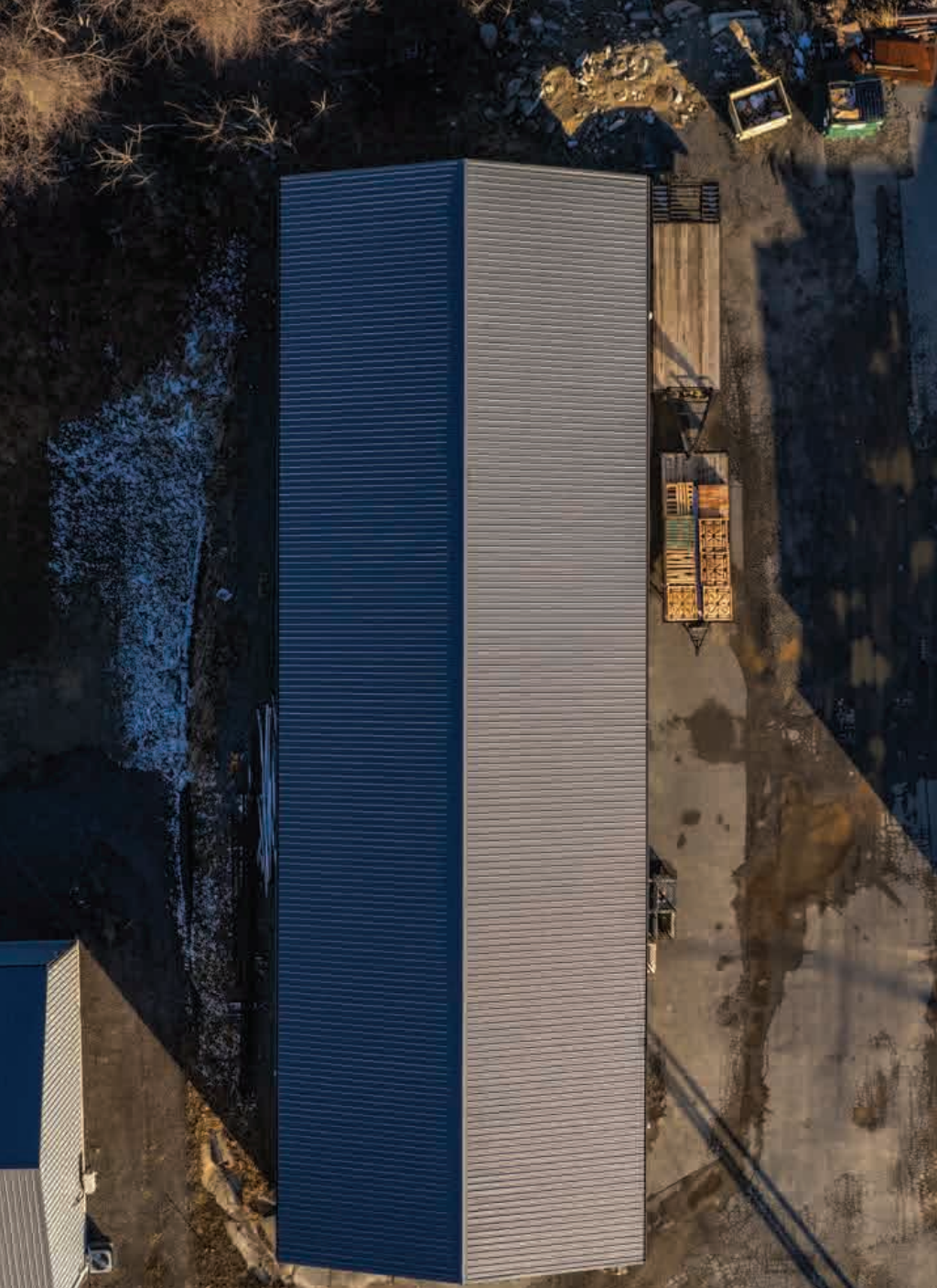
Building 247: View from Above.
