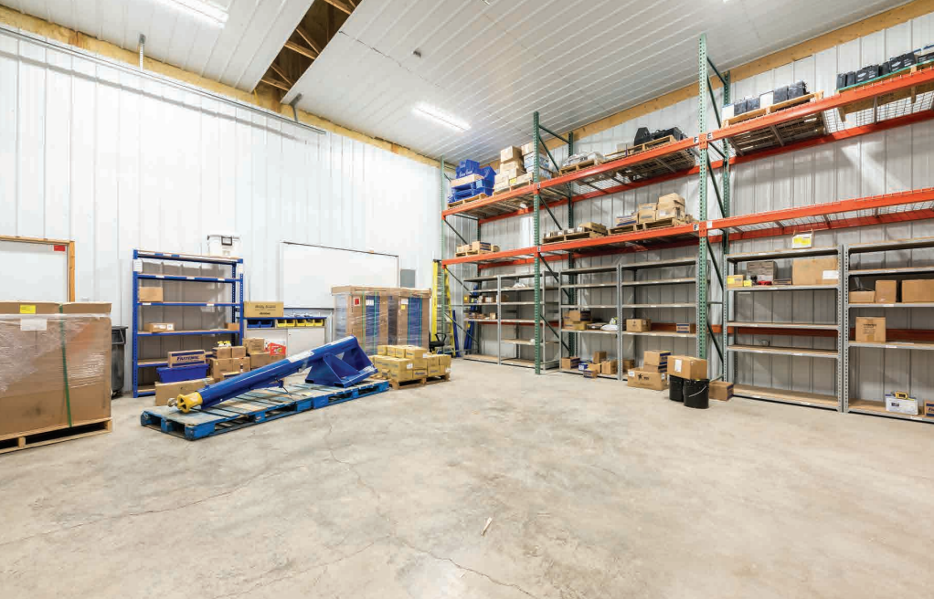
Side Industrial Area.
