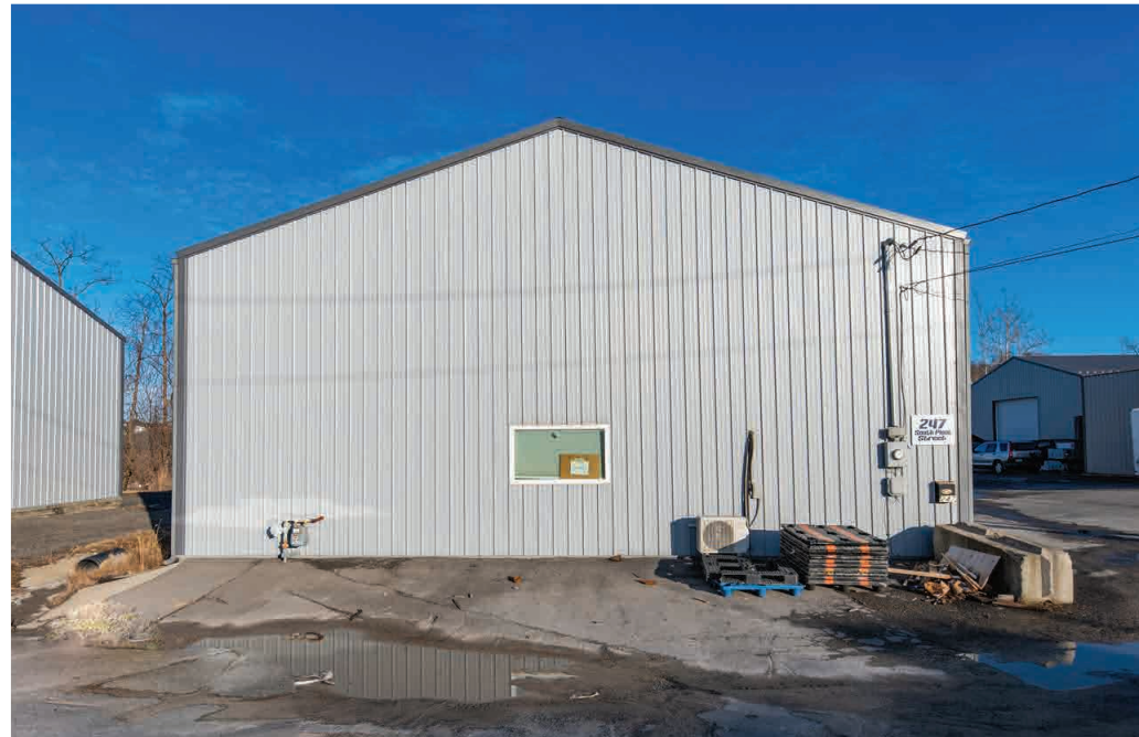
Building 247: View from the Main Road.
