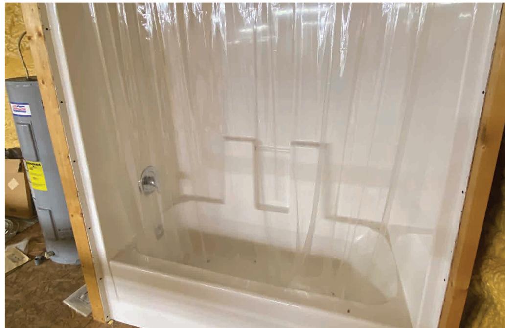
Building 247: Mezzanine Shower.
