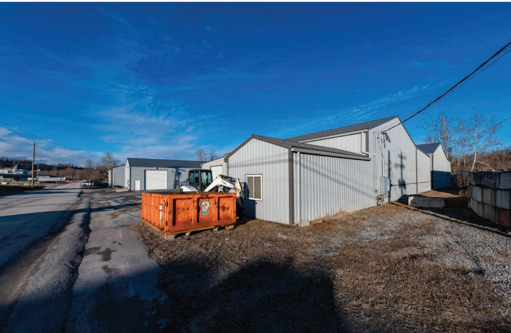
Building 249: Back Building.
