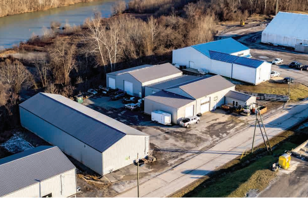
Aerial View of the Property Facing Southeast.
