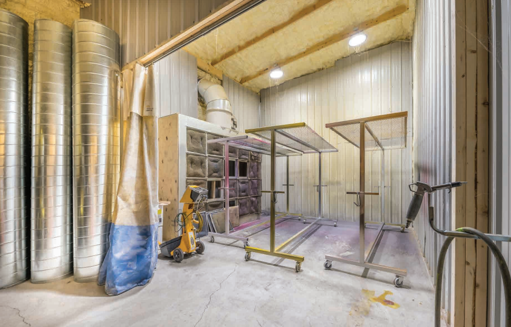
Back Building, Back of Storage.
