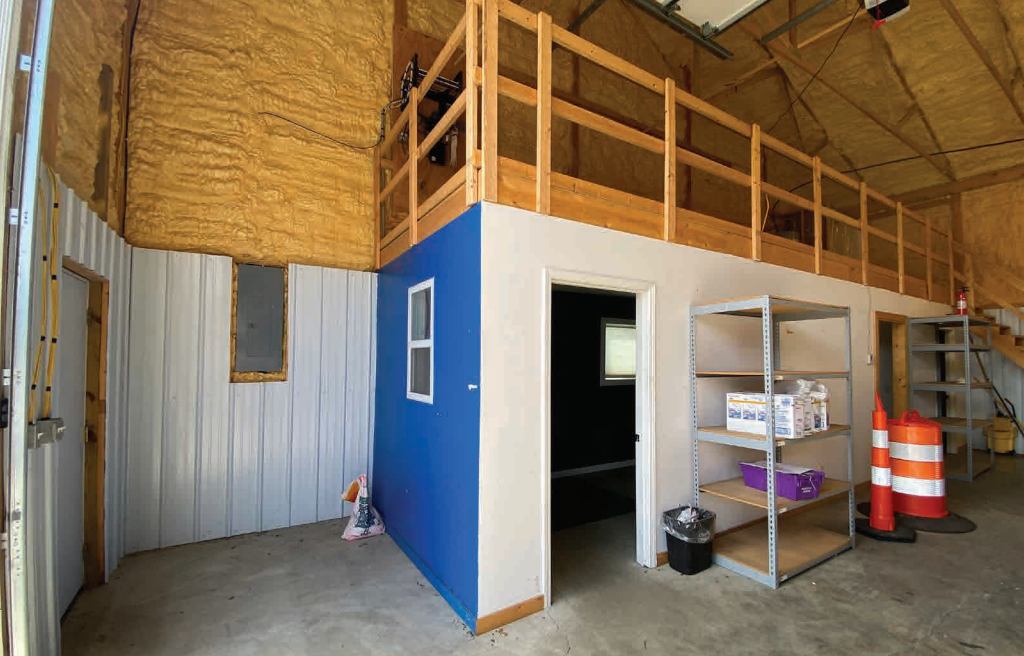
Building 247: Office and Mezzanine.
