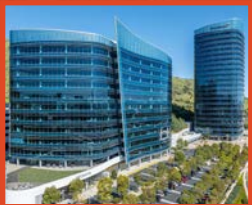
ONE & TWO TOWER PLACE
