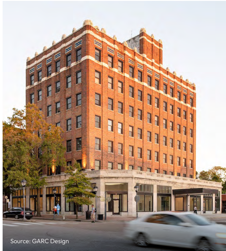
Figure 14 505 Washington Street - Professional Building
