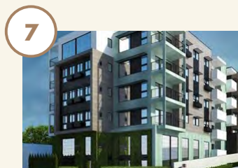
3917-19 Louisiana St - U/C 23 units
