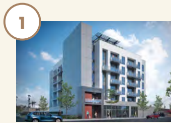
Vadara West - U/C 50 units
