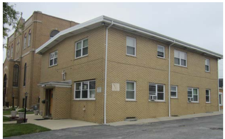
SIDE OF RECTORY
