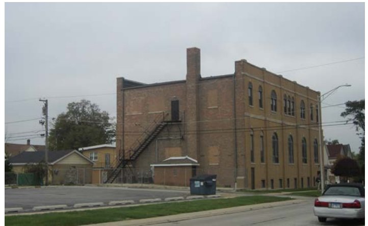
BACK OF CHURCH BUILDING
