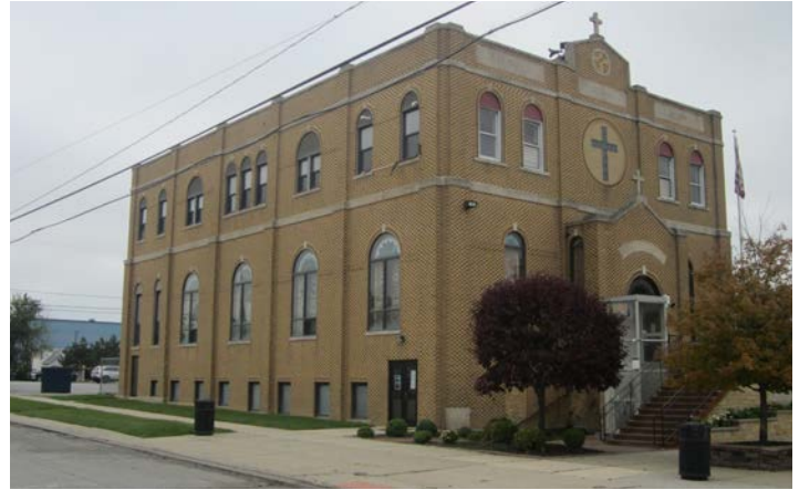
SIDE OF CHURCH BUILDING
