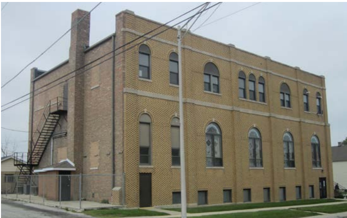
SIDE OF CHURCH BUILDING
