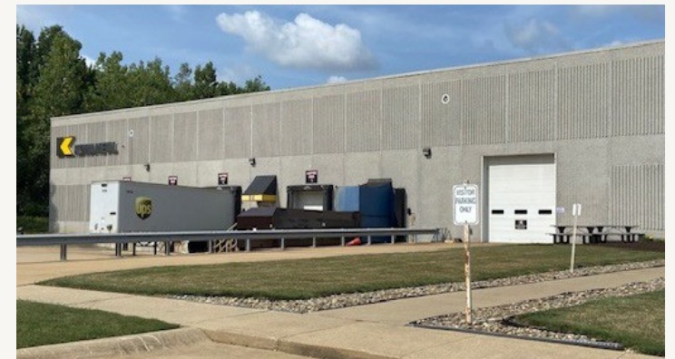
Service area and compactor
