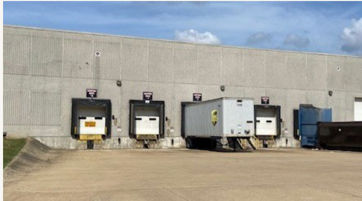
Precast exterior and dock line
