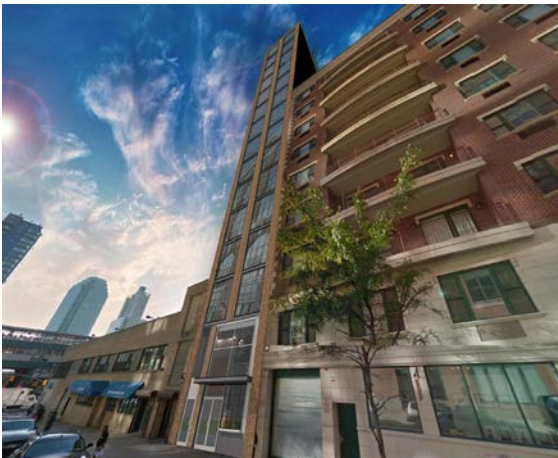
41-32 27th Street - Steel Haus 44,581 Sq. Ft., 46 Units
