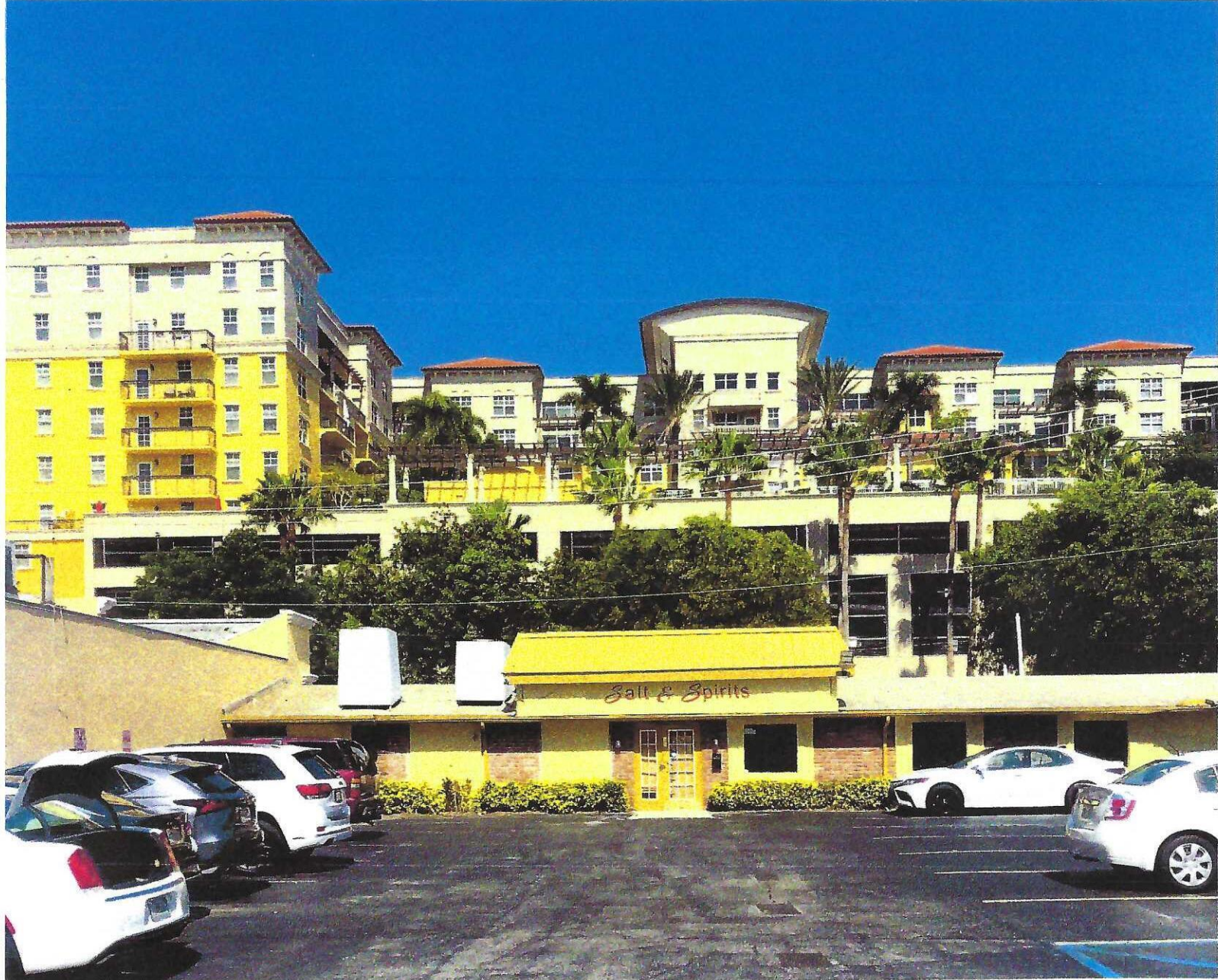
VIEW TO THE EAST ROYAL PALM PLACE APARTMENTS
