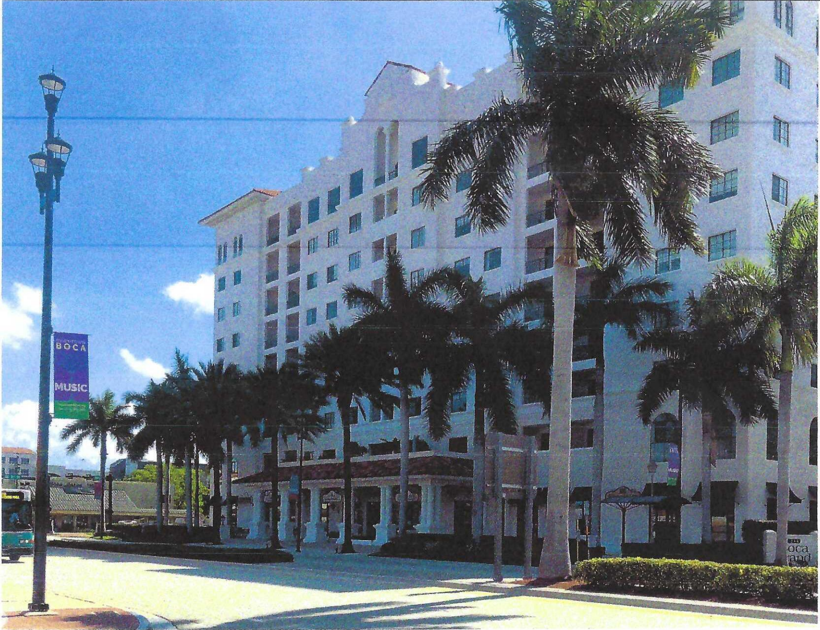
VIEW TO THE SOUTHWEST THE BOCA GRANDE CONDOMINIUM
