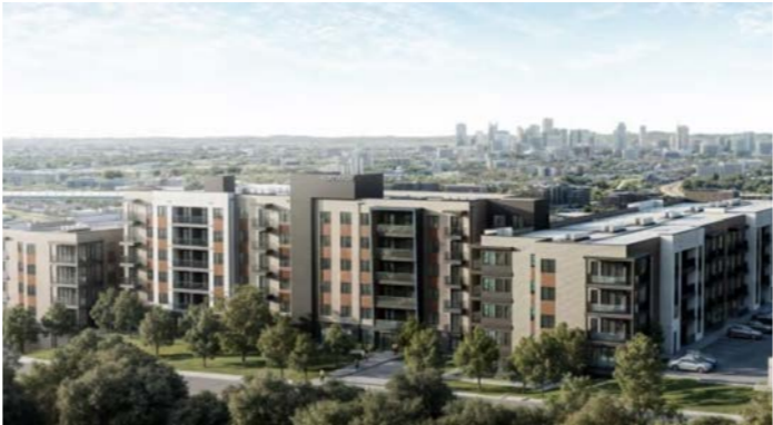
NORTHVIEW 254 UNITS (UNDER CONSTRUCTION)
