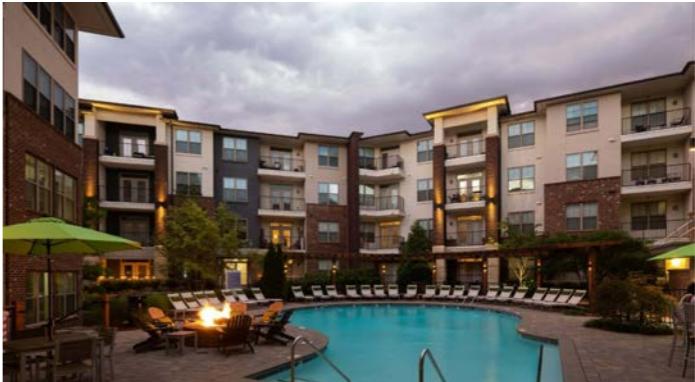
ONE METROCENTER 320 UNITS (2015)
