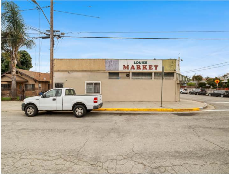
Front of Retail Store and Apartment Entrance on Left
