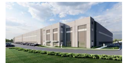
6 | WEST END LOGISTICS CENTER
