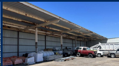
LARGE CANOPY STRUCTURE
