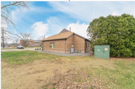
View of side of home featuring brick siding
