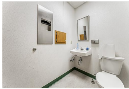
Bathroom with toilet and baseboards
