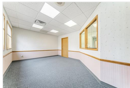
Spare room featuring a drop ceiling, wainscoting, and visible vents
