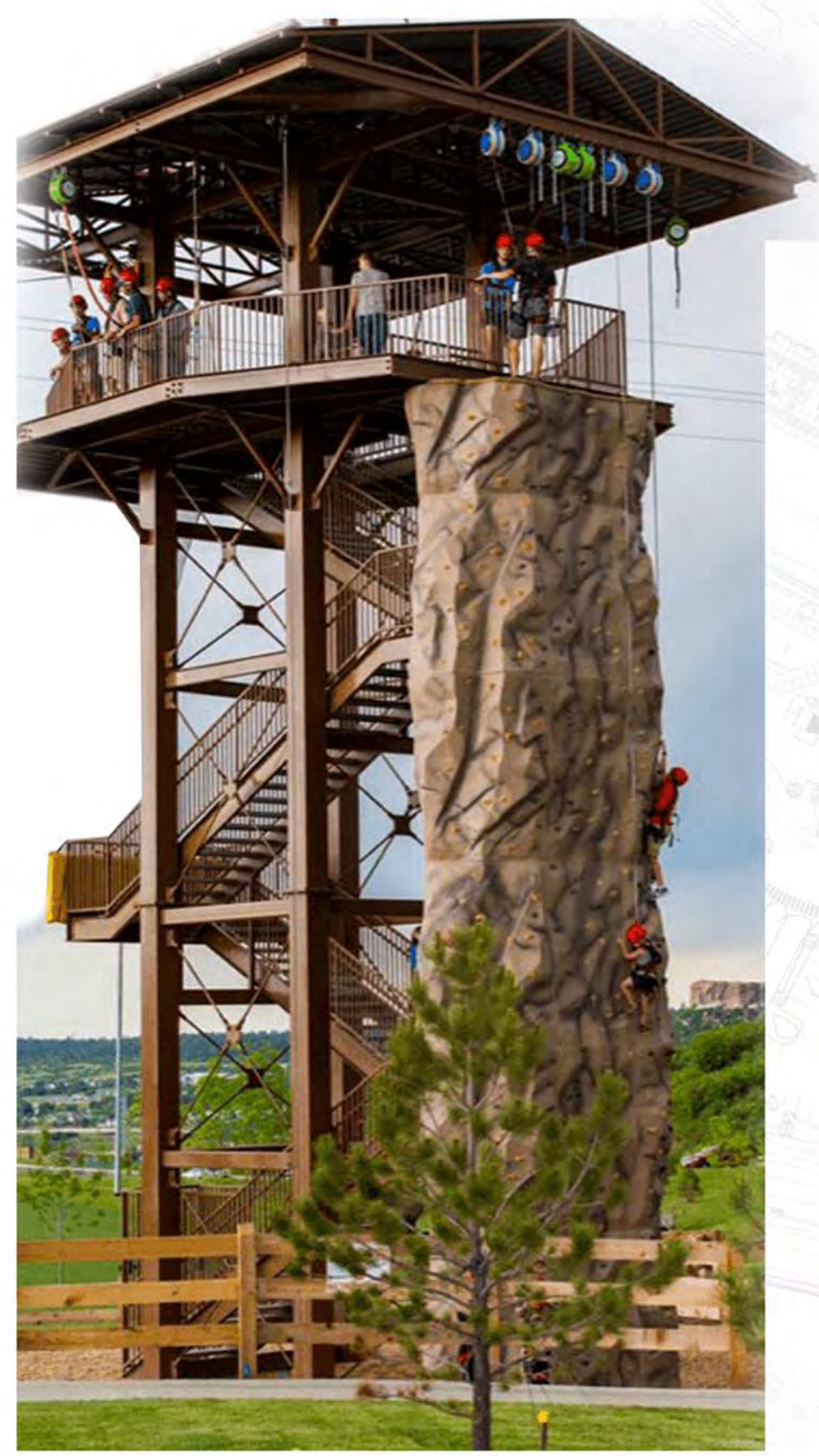
Zip Tower and Climbing Wall
