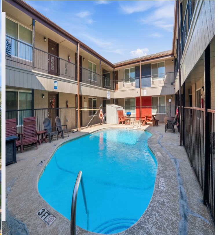
Inside Corridor Area
