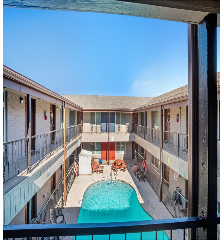
Inside Corridor Area
