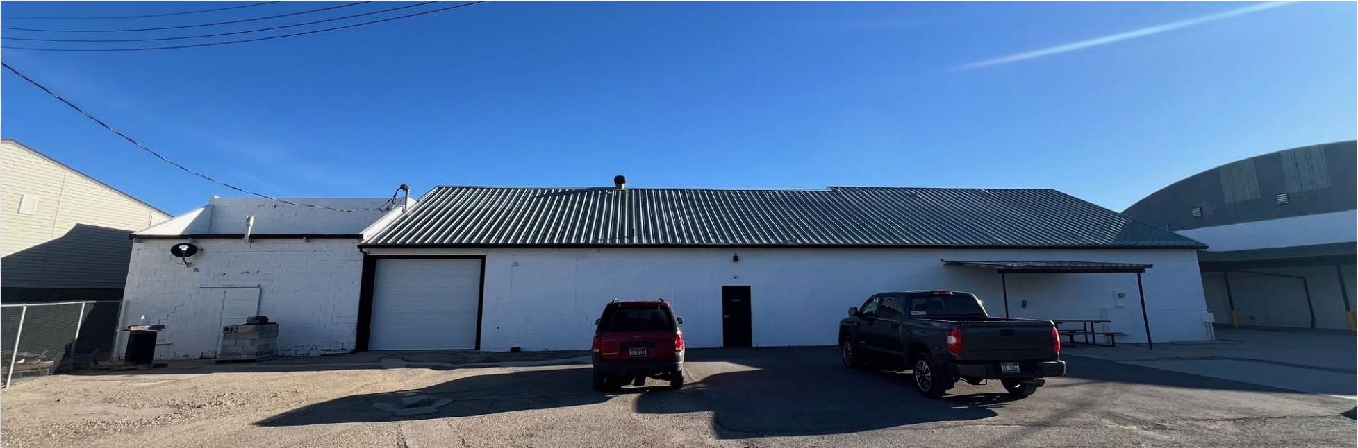
UNIT 3 EXTERIOR SIDE
