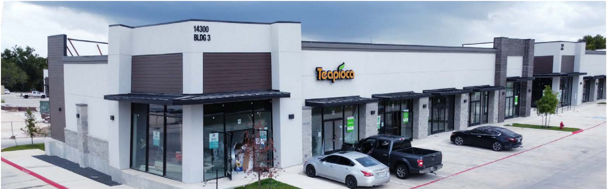
CONSTRUCTION PROGRESSION SEPT 2024
