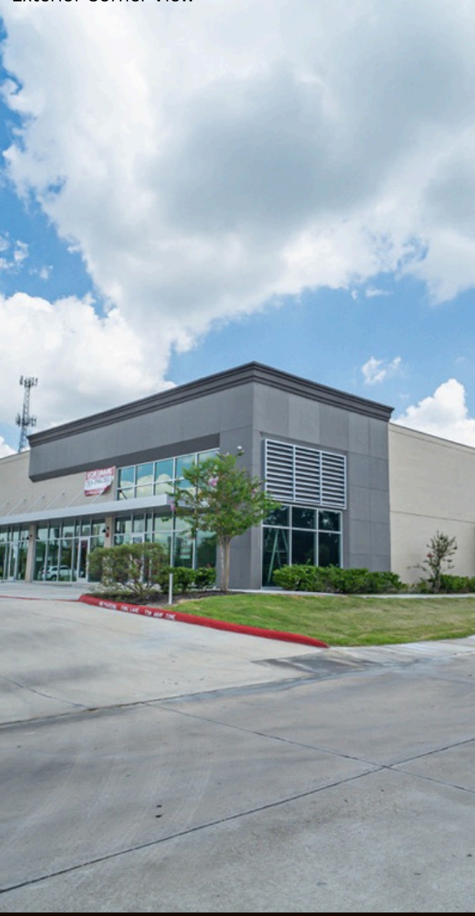
Exterior Corner View
