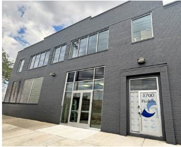
Rear Along Perkins Avenue
