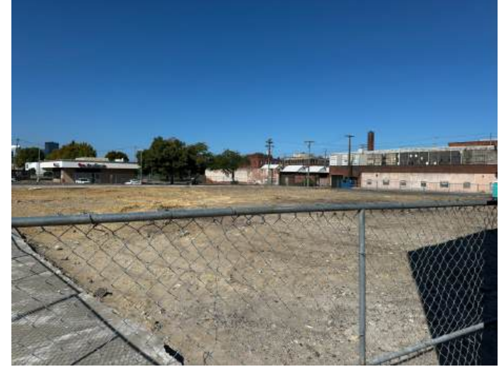
Parking Lot Under Construction
