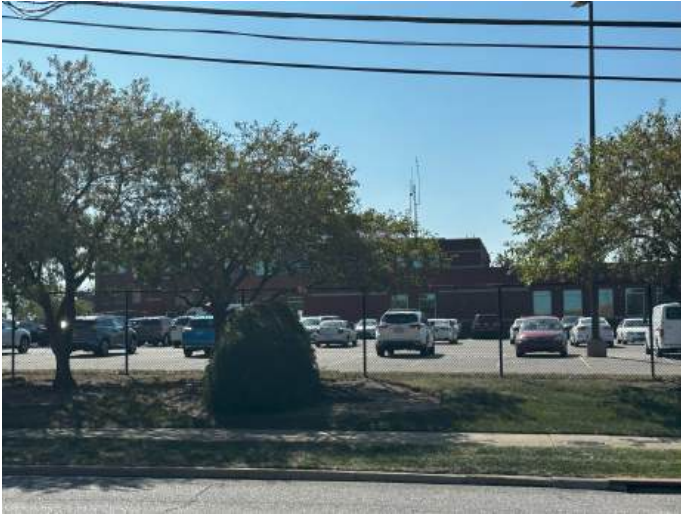
Leased Parking Lot
