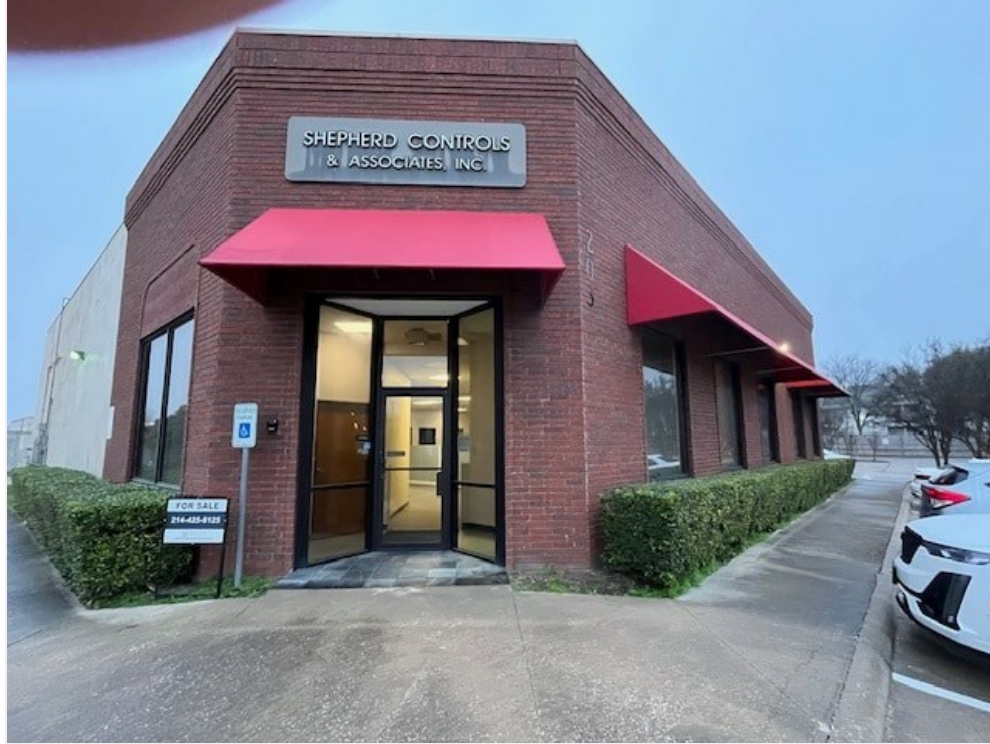
Exterior Front Entrance
